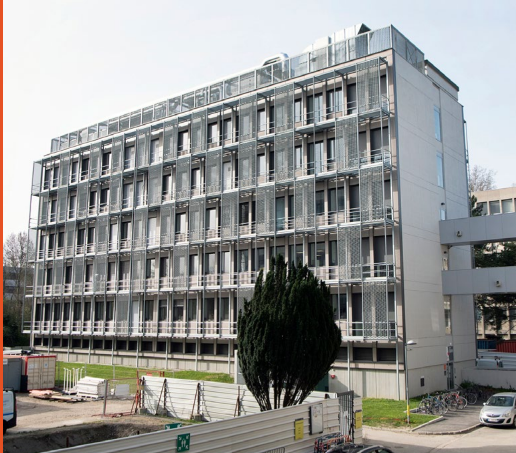
Renovated Dubois building (LyonTech - la Doua Campus)
