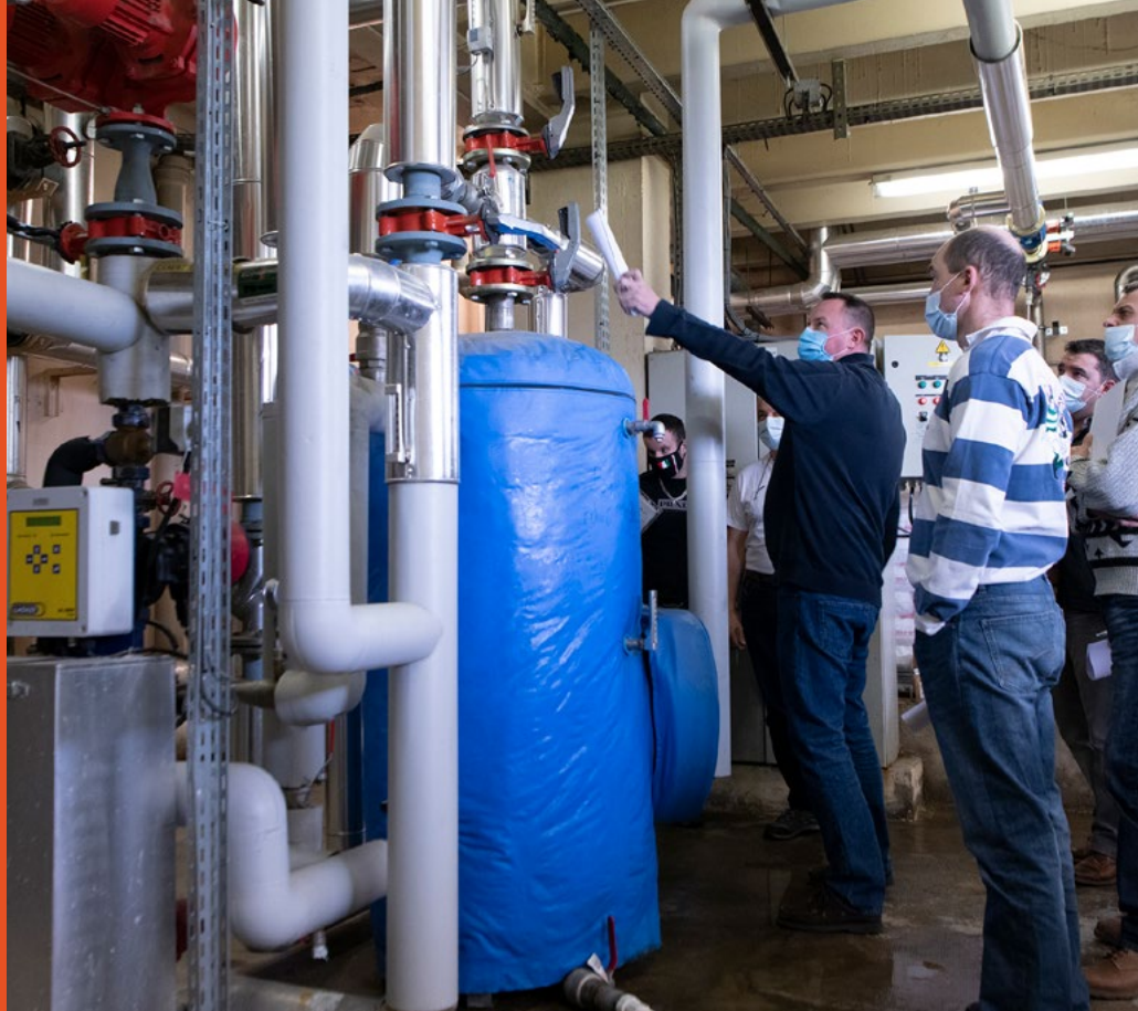
Training on the prevention of the risk of infection linked to the environment and hot water network
